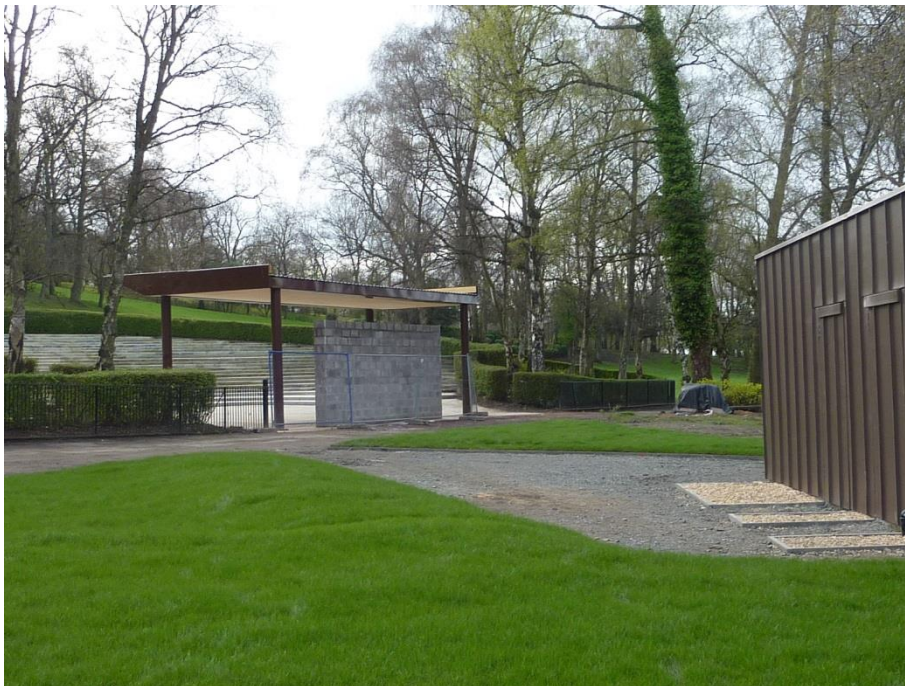
Canopy and facilities block under construction, 2014
